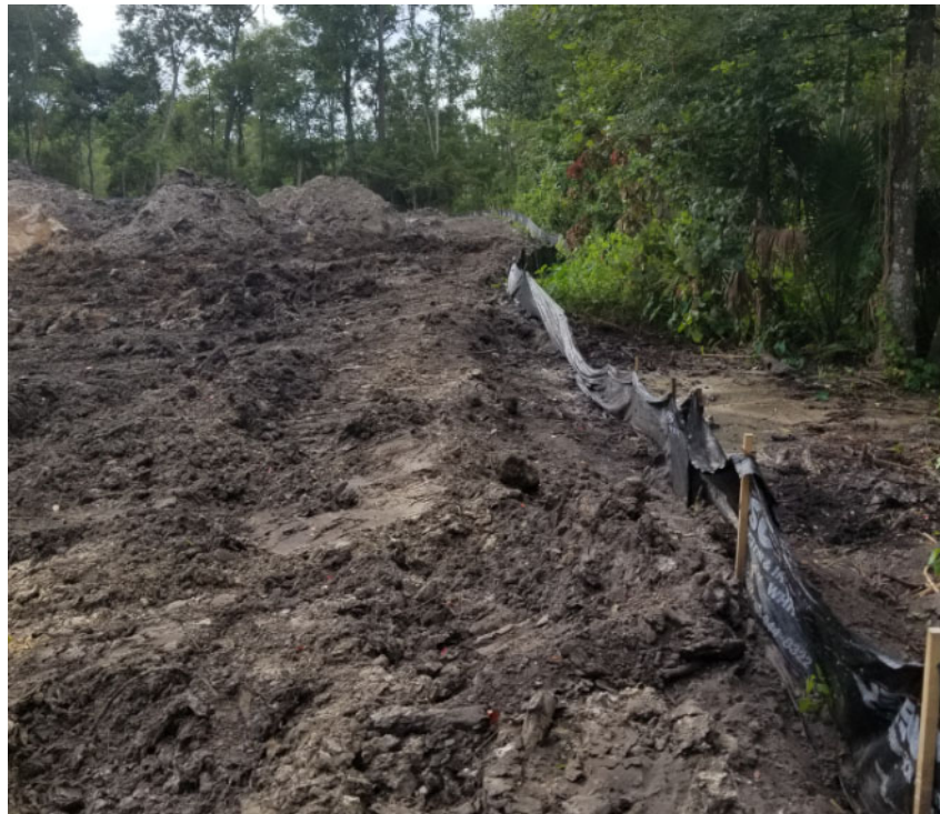
Photo 9: 7-19-2021: Silt fence along western Conservation Easement boundary.
