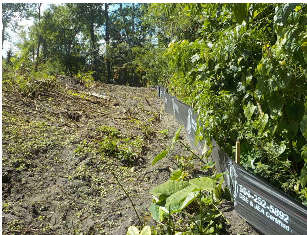
Figure 2: 6-8-2021: Silt fence on western Conservation Easement boundary.
