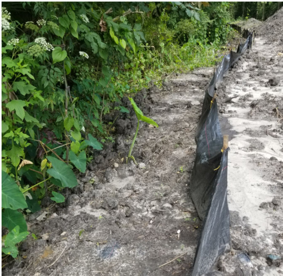
Figure 4: 6-29-2021: Muck beyond silt fence on western Conservation Easement boundary.
